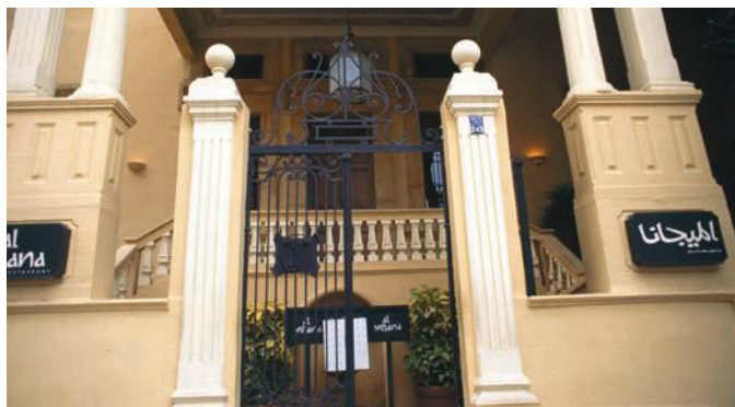
b These gates are made of iron. Iron can easily be moulded into different shapes.
