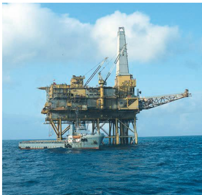
Figure 6.7 Oil production in the North Sea.
