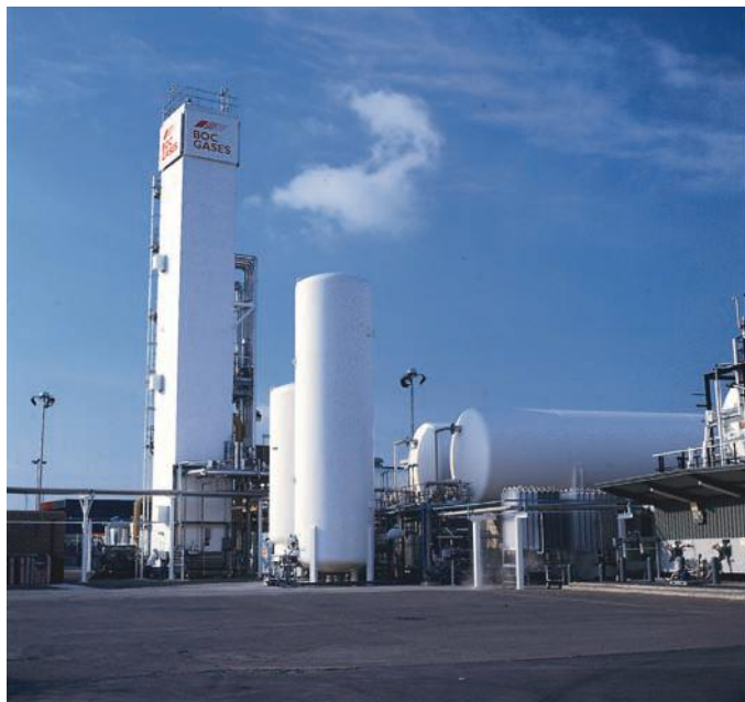
b Gases from the air are extracted in this fractional distillation plant.
