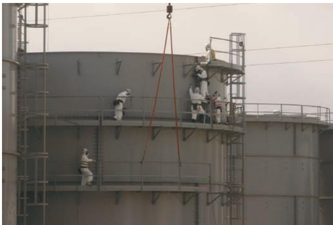
Figure 6.13 Workers wearing protective suits and masks at the Fukushima power plant.
