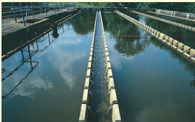
Figure 2.39 Water is treated to remove suspended solids by the addition of aluminium sulfate.
