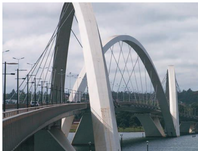
Figure 13.6 This bridge in Brazil uses reinforced concrete.
