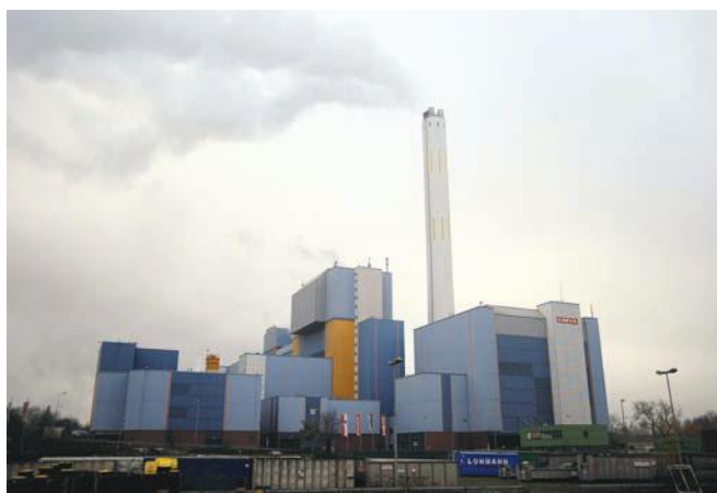
Figure 14.23 A plastic incineration plant in Germany.
