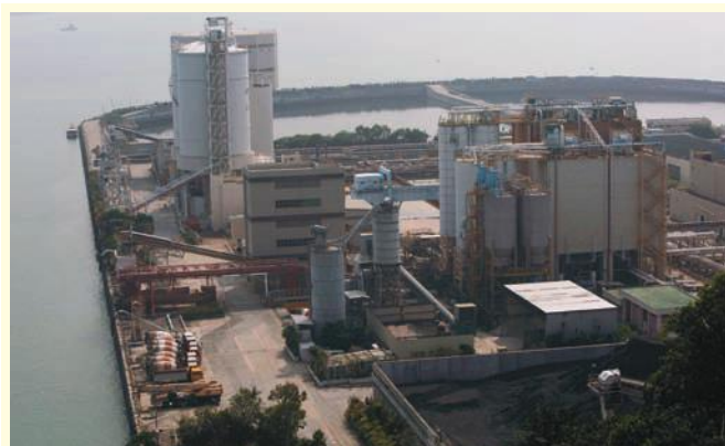
Figure 6.9 A Hongkong Electric Co. Power Station, Hong Kong, China.
