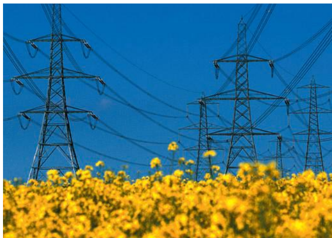
Figure 5.16b Due to the high density of copper and its cost, steel-cored aluminium cables are used for electrical transmission through national grids.
