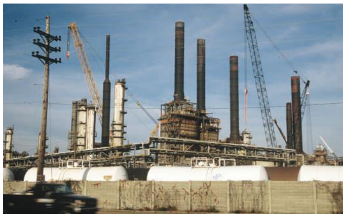
a Fractional distillation unit for crude oil.
