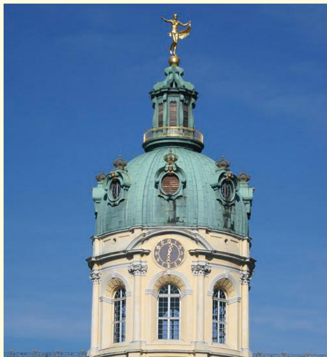
Figure 10.26 Verdigris soon covers copper roofs in exposed environments.
